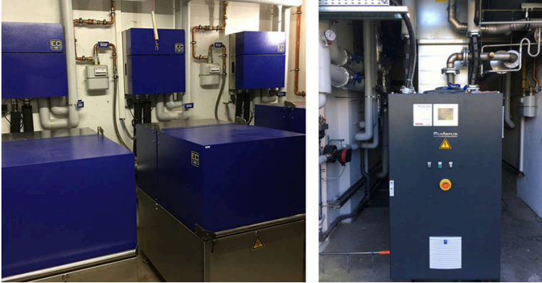
Fig. 2: CHPs of the electroplating company.
